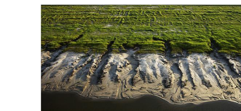
Two kinds of overtopping-induced damage
