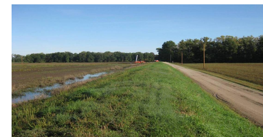
Resilient, overtopping resistant clay levee
