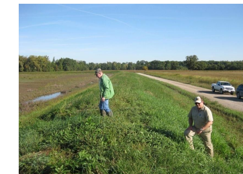
Resilient, overtopping resistant clay levee
